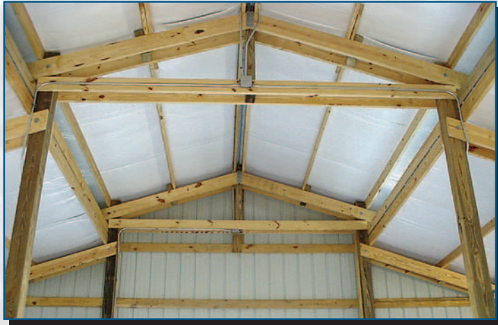
Wood Purlin on Wood Truss
